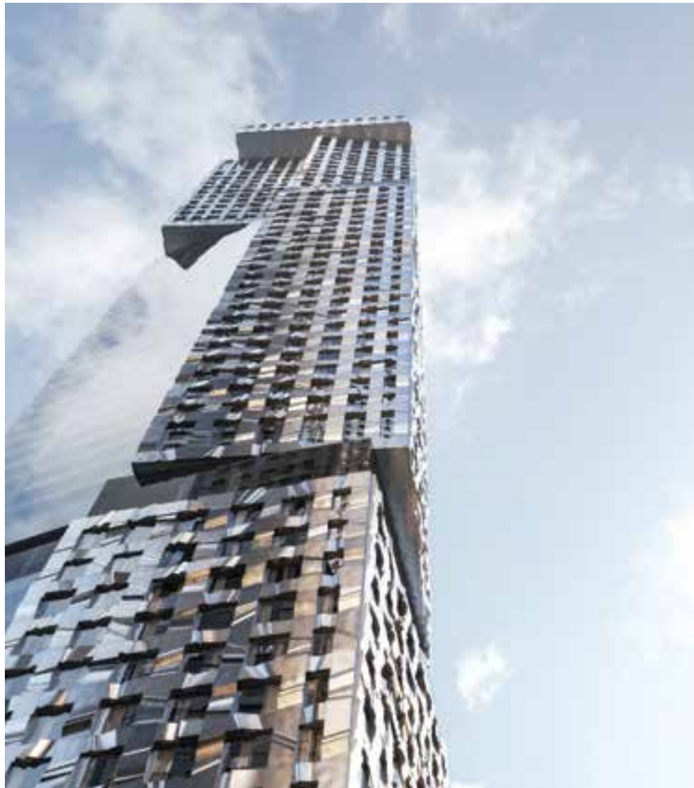
East Tower Façade
